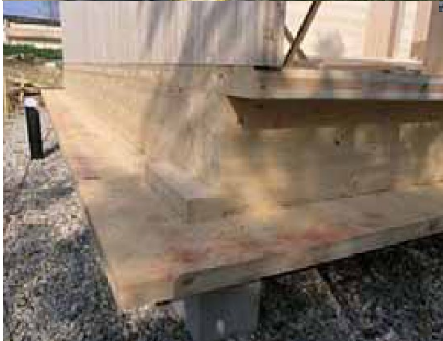
S-House Austria: single foundation points, no sealing, but still compaction of soil
