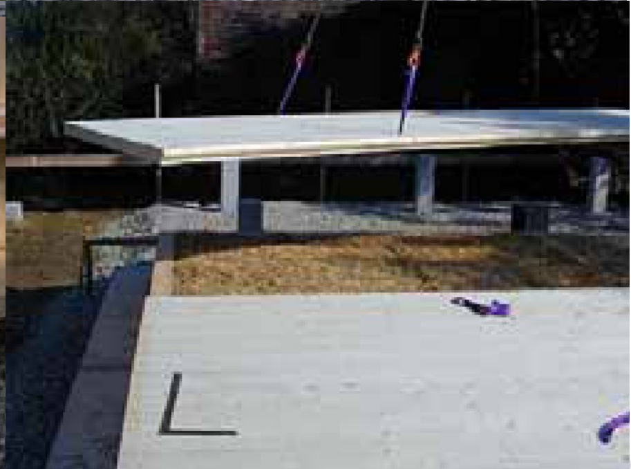
S-House Austria: single foundation points, no sealing, but still compaction of soil
